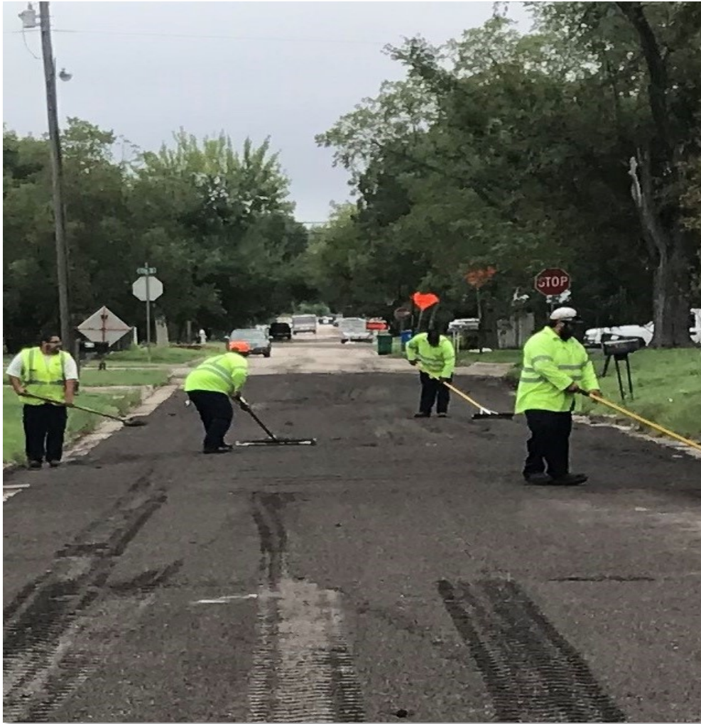
Street Crew Raking Asphalt for Level-Up Program
